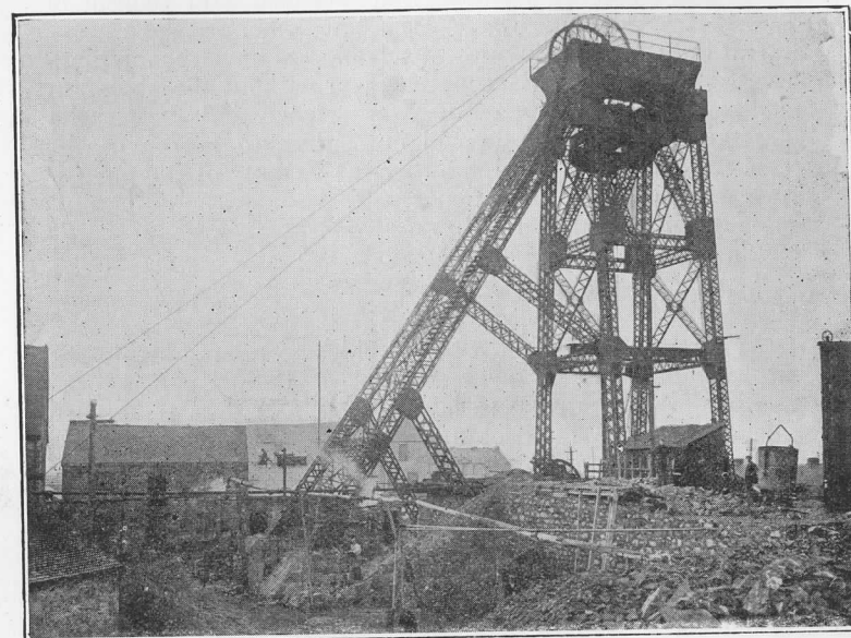
TYPICAL STEEL HEADGEAR.
